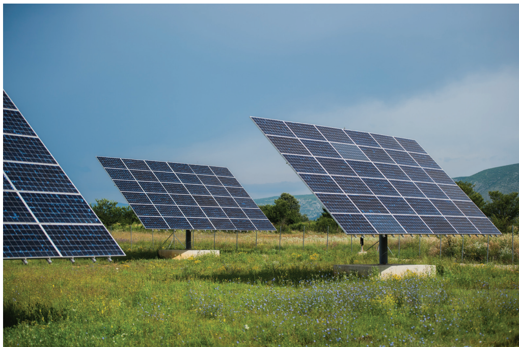
Tomings' solar panels are perched on concrete poles and are synchronized with the sun to produce more electrical energy. (Photo:CIN)
